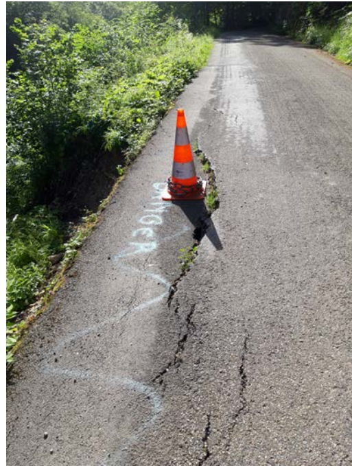
Figure 4 : Fissurations importantes
